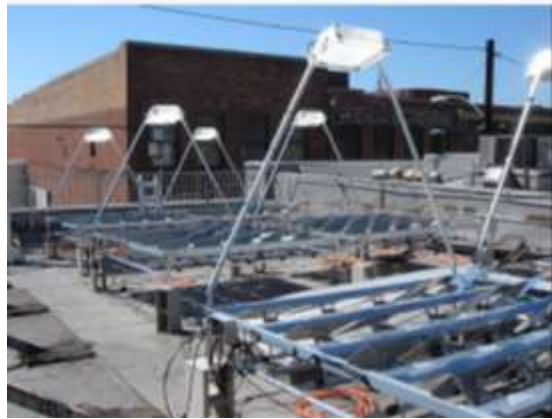
Fig1. Reflective mirror based solar trackers (Image source: Wikipedia)
